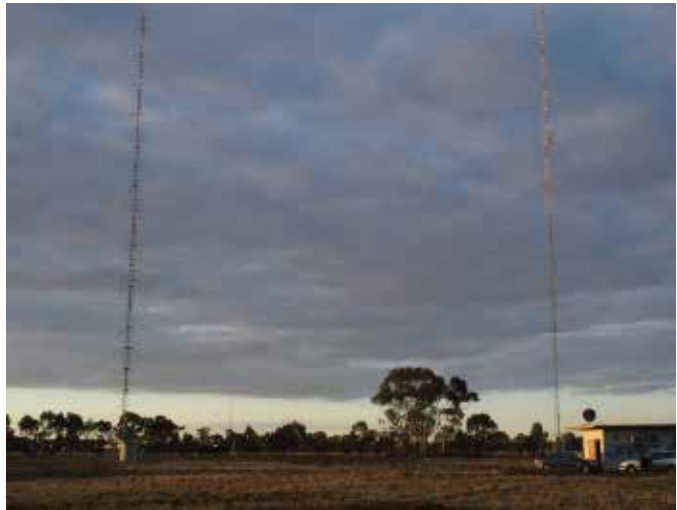
3CR transmitter site, Werribee
